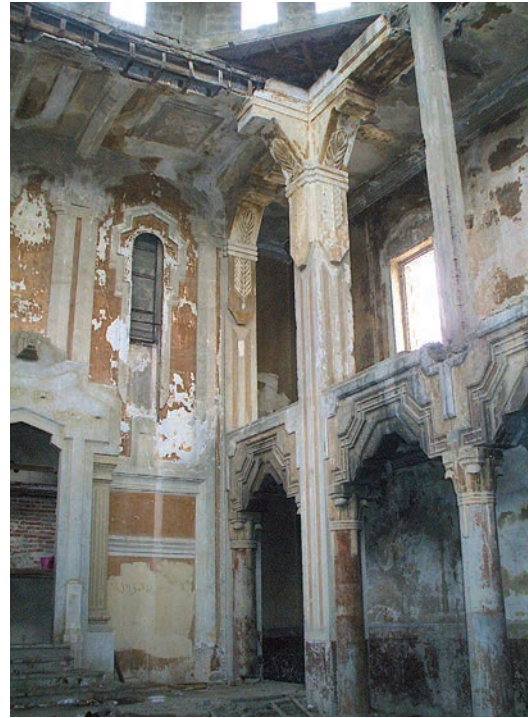
Fig. 6 - View of the interior space of the Synagogue. (Author's photo, 2008). Fig. 7 - View of the interior space of the Synagogue. The triangular corners of the new octagonal slab, supporting the hemispherical dome, and the new plain pillars, different from the original ones, are very evident. (Author's photo, 2009).
