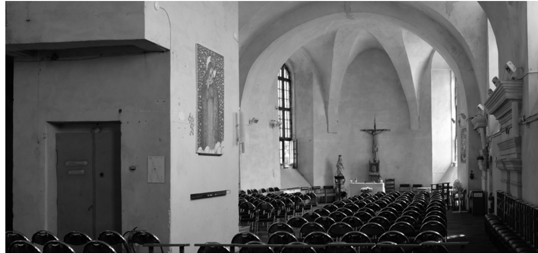
Fig. 4 - Panoramic views of the first and second floor, where the Soviet structures are clearly visible..
