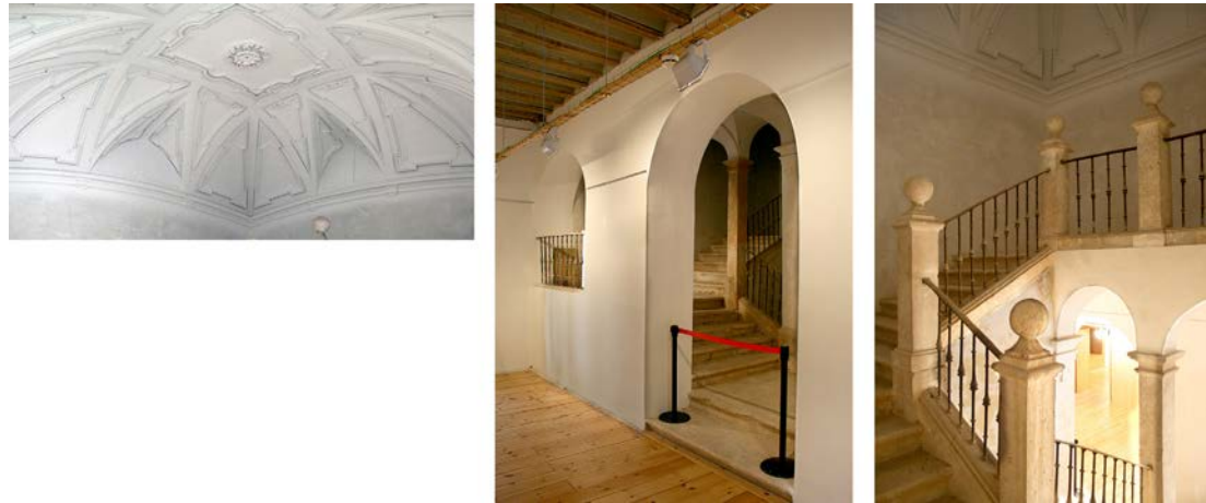
Fig. 15 - Main staircase of the Goyeneche Palace in Nuevo Baztán (Madrid). Author.
