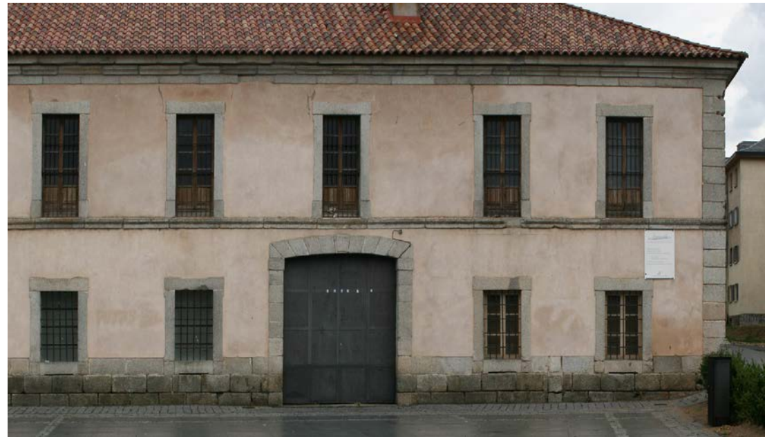
Fig. 6 - Royal Glass Factory of La Granja (close reference), building in 1770 by architect Díaz Gamones. Author.
