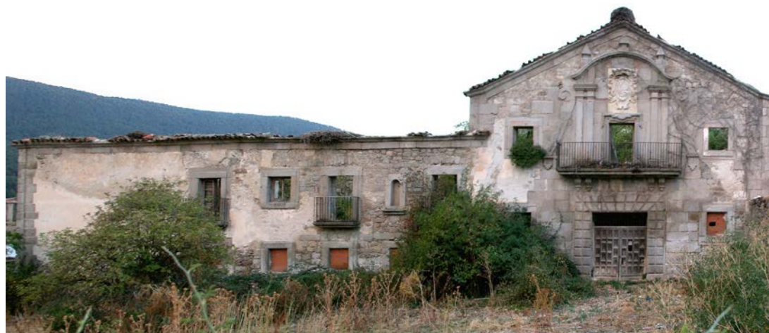
Fig. 2 - Main façade of the Perales shearing building in El Espinar (Segovia). Author.
