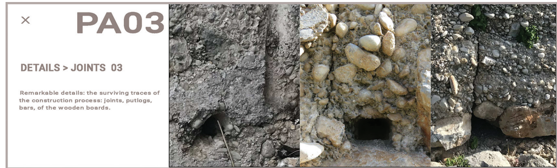
Fig. 11 - Example of an informative panel detailing the traces of the wall construction process.
