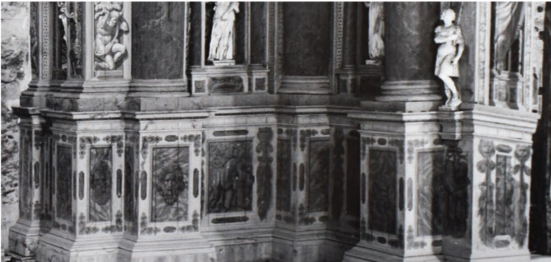
Fig. 4 - Detail of the original proscenium decoration (pedestal). Photograph from Pinazzi private collection
