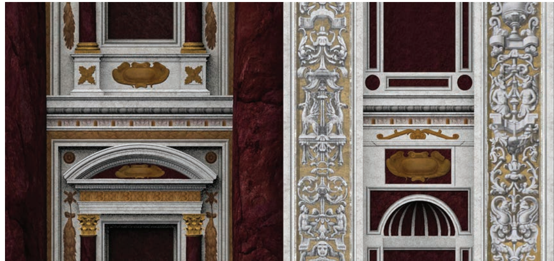
Fig. 6 - Detail of the 3D textured model of the proscenium with a reconstruction of elements clearly documented in the photographs taken before the destruction (grotesques).
