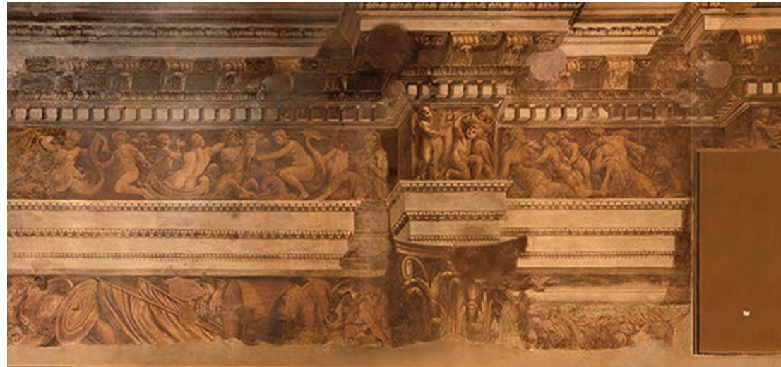
Fig. 5 - Detail of the orthophoto of the fresco placed on the back wall of the hall (entablature).
