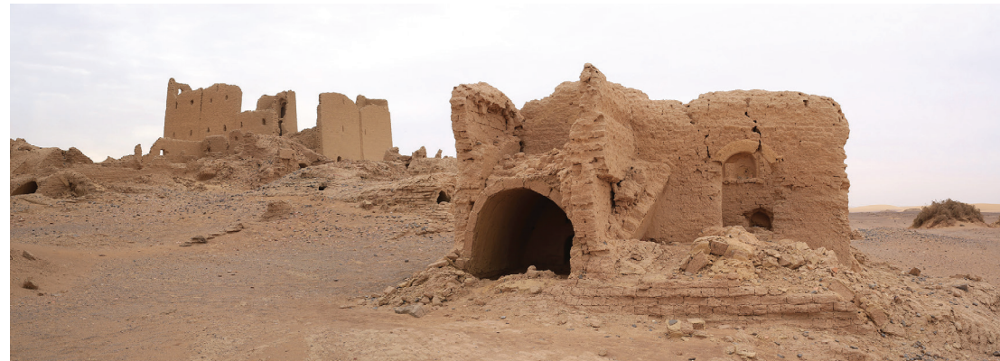
Fig. 3 - Panoramic image of the site seen from north, with the domestic Unit A in the forefront and Fort in the background.
