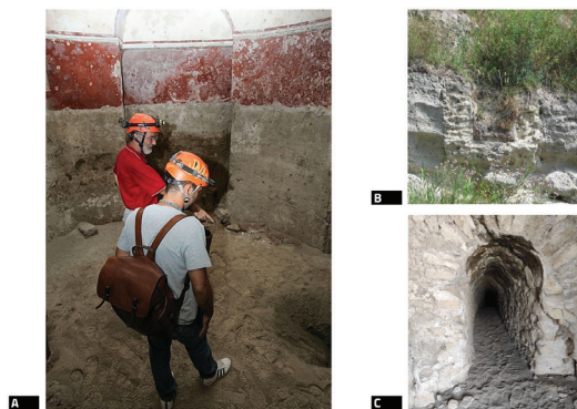
Fig. 7 - In the picture: A. Photographic survey; B. Photogrammetric survey; C. Dense Cloud; D. Material Survey; E. Comparison and updating of the survey filed at the Municipality municipality of Bacoli.
