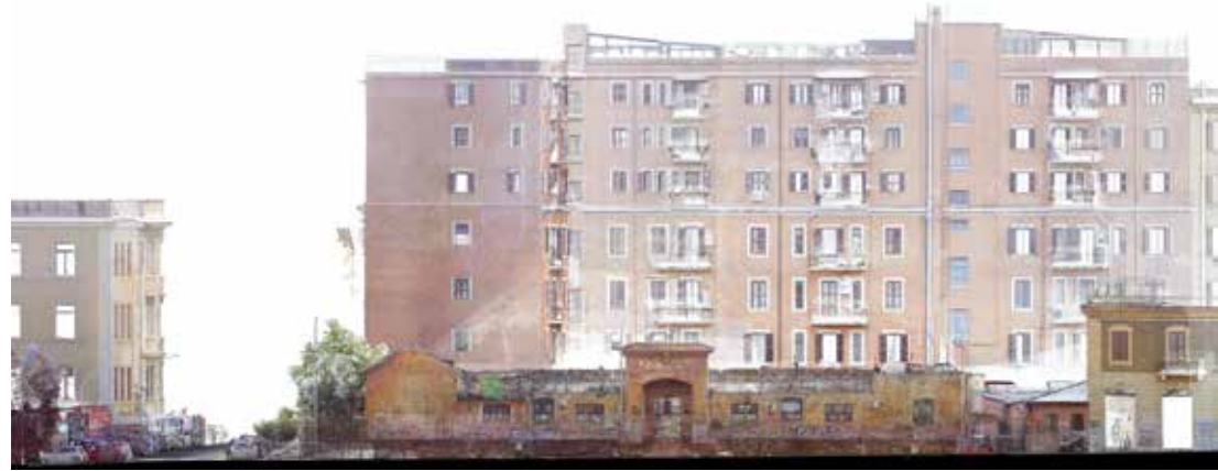
Fig. 18 - Orthophotoplan of the Ex-Filanda obtained from a point cloud. The point cloud was created through an integrated instrumental survey, using laser scanner technologies and drone shooting.
