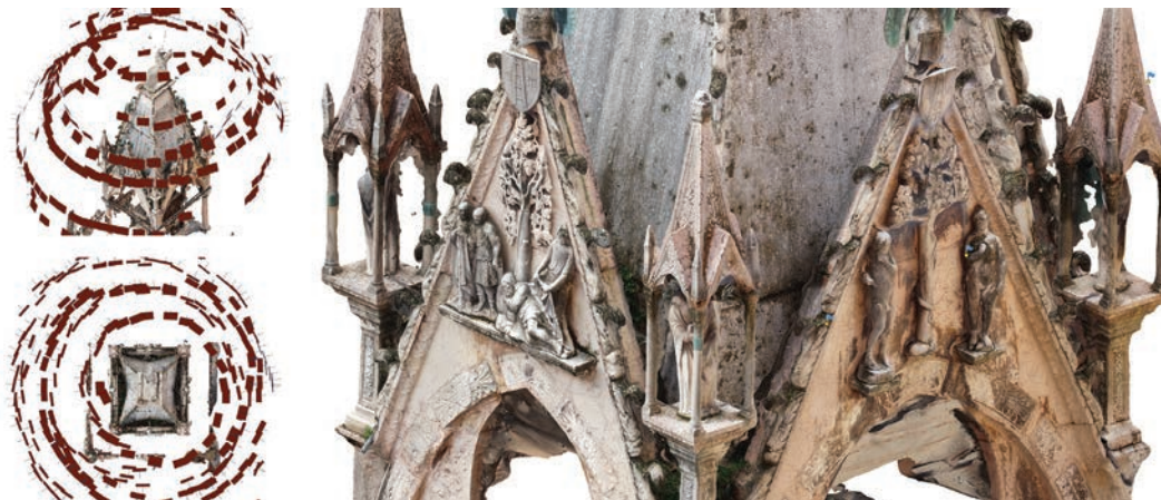
Fig. 6 - Detail of the mesh model elaborated from UAV photogrammetry.
